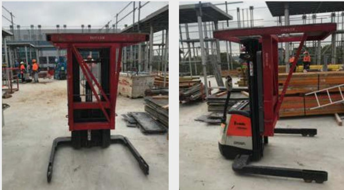
Super Destil formworks are hydraulically lifted, lowered and horizontal repositioned through the use of a standard handling unit combined with an applied special metal frame. The lifting appliance, by just one man work, allows formworks to be moved in a safe and fast way.
